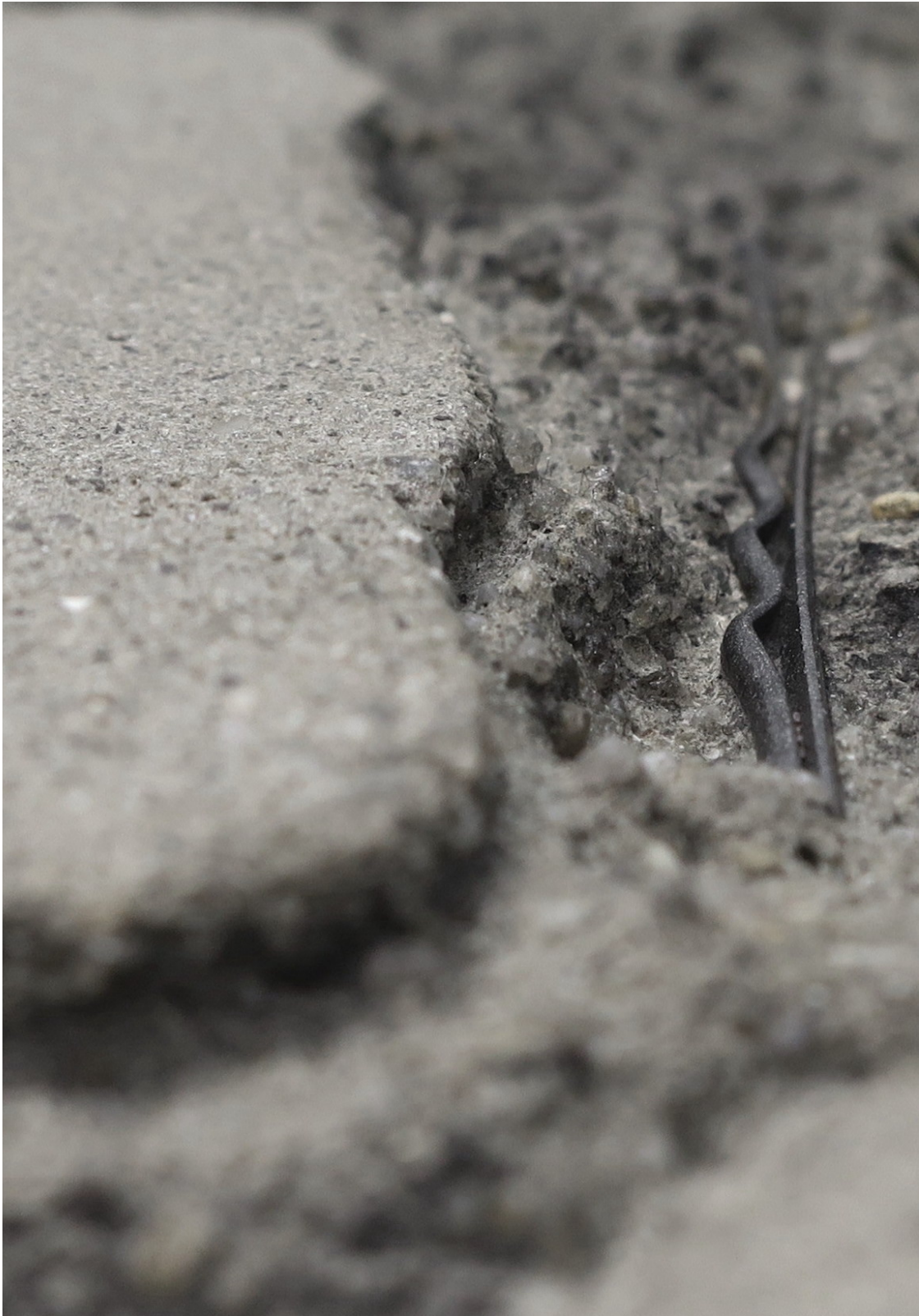
The Invisibles , betong, stål, detalj, 2024
