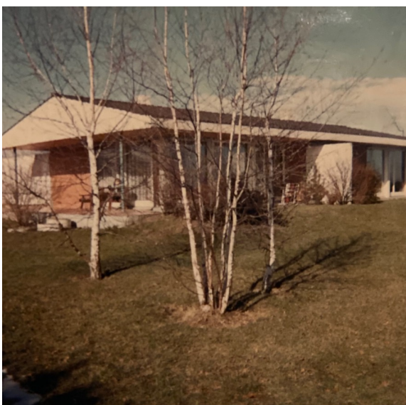
K's residence (affordable villa by Le Corbusier)
