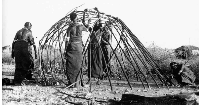
Figure 4 Armature of a Rendille Tent. The frame of the armature in the process of assembly. Note the sturdy straight poles of the lean-to entrance which are not buried but rest directly on the ground. The woman on the bottom right is securing these with rocks. Photo by Anders Grum, Keenya, 1975
