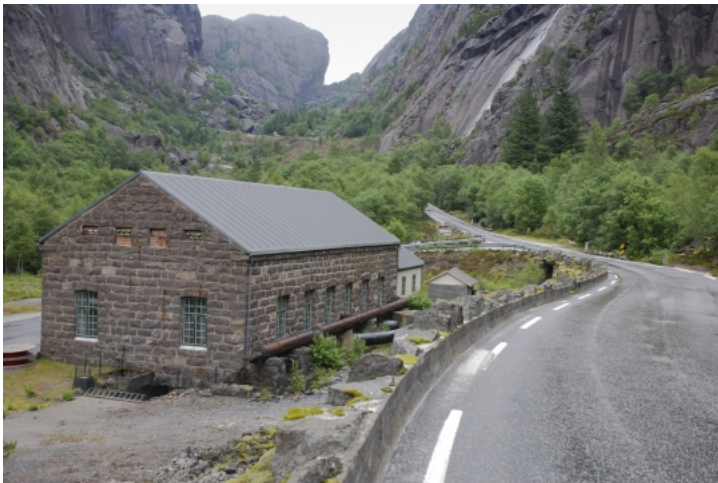
Fig. 3. Nedre Hellenen hydropower plant from 1907. Jan Ove Grastveit.
