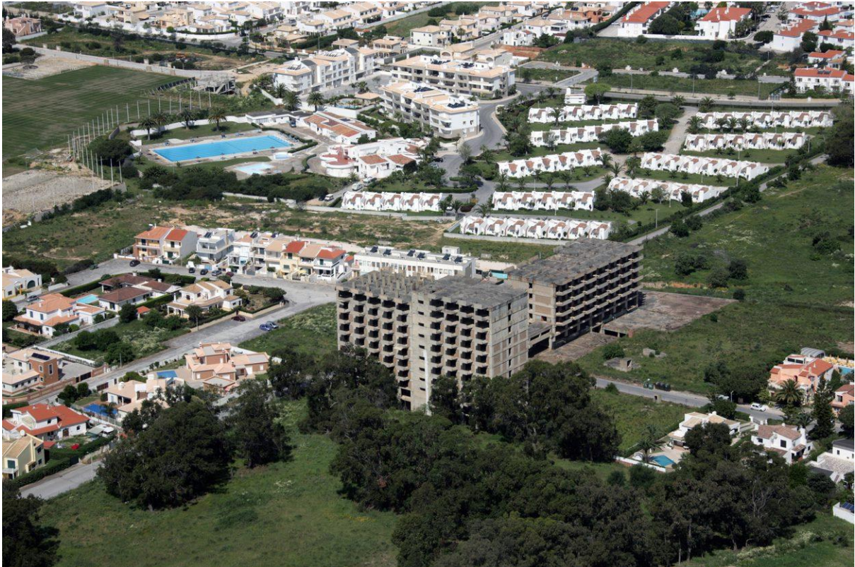
Image4 – “As Torres” That is how the locals call these abandoned buildings in Lagos/Portugal
