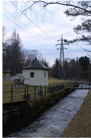
Hammeren hydro-electric plant Photo: Unn Yilmaz/NVE
